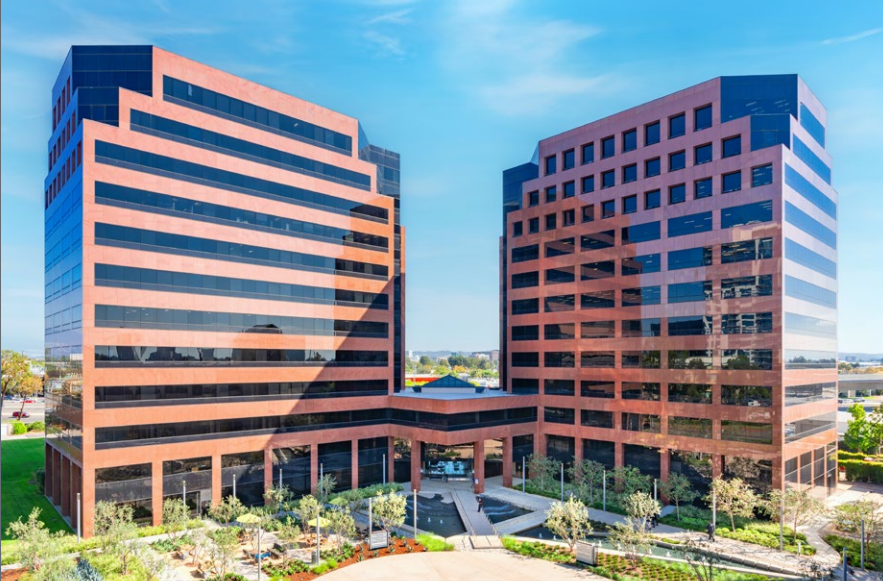
GRIFFIN TOWERS • Santa Ana, CA • Acquired: April 2023
